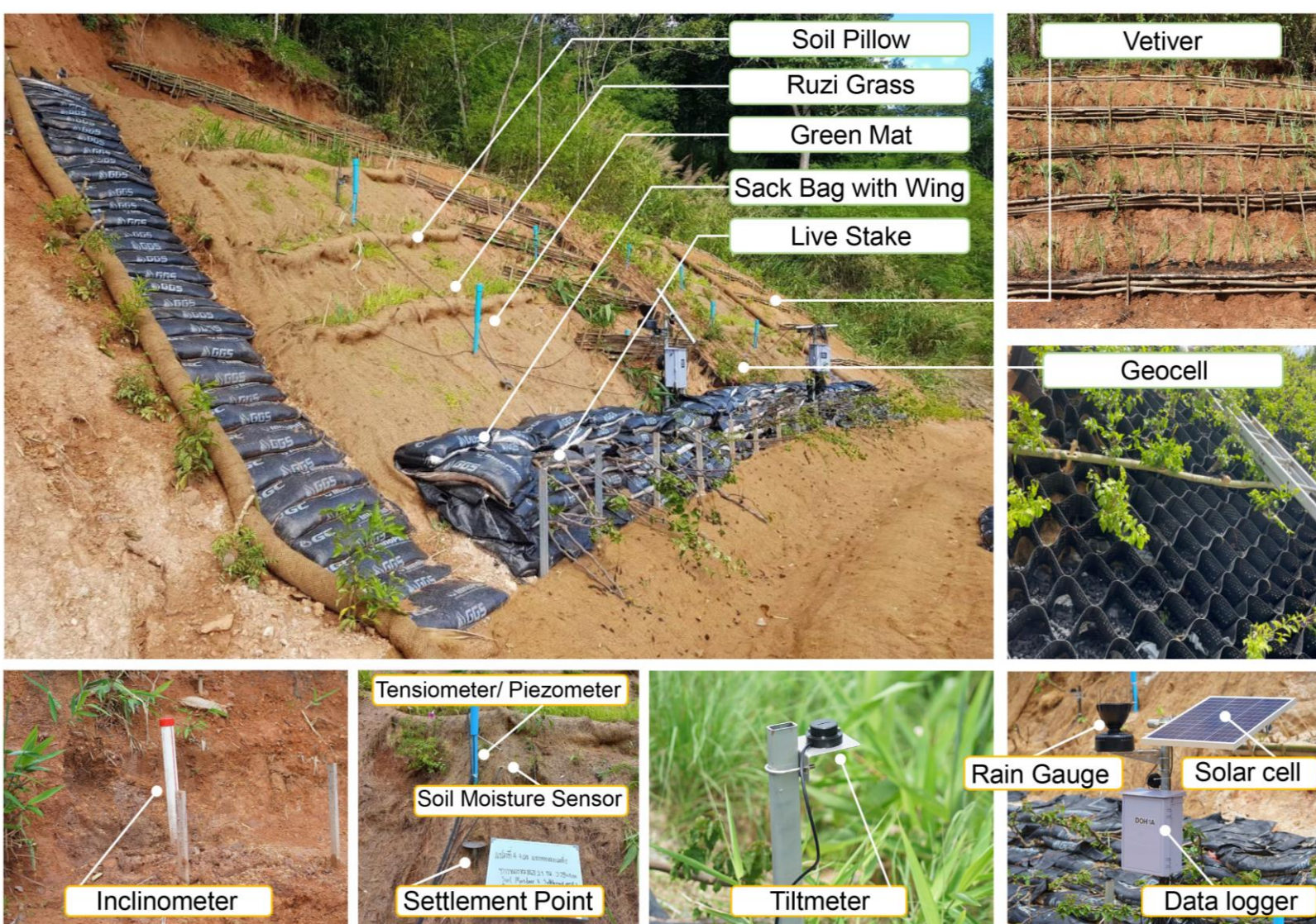
Figure 5 - Photographs of test section 4.
